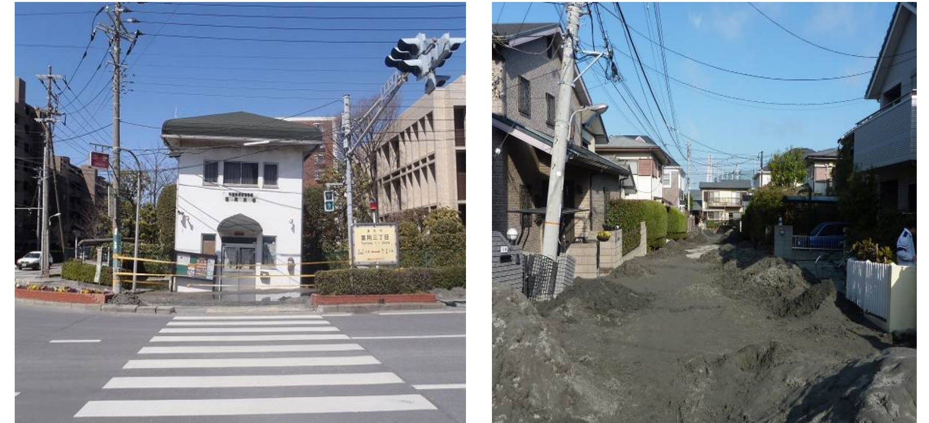
Fig. 1. Road condition of main road and residential road after the Great East Japan earthquake
