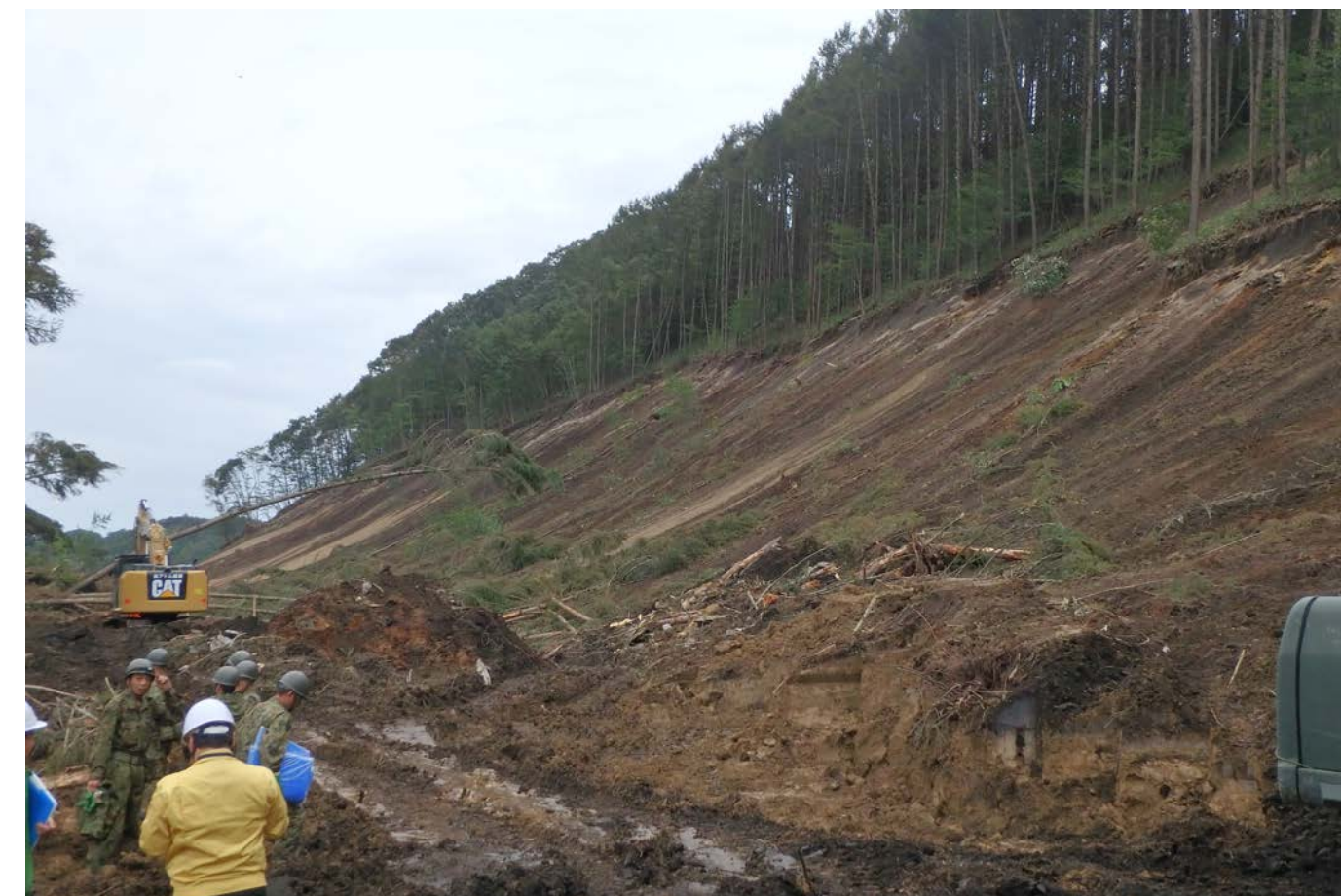
Fig 1 – Landslide in Atsuma Town
